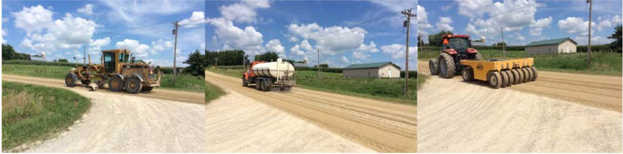
Figure 44. Chloride treatment at Goodhue County
