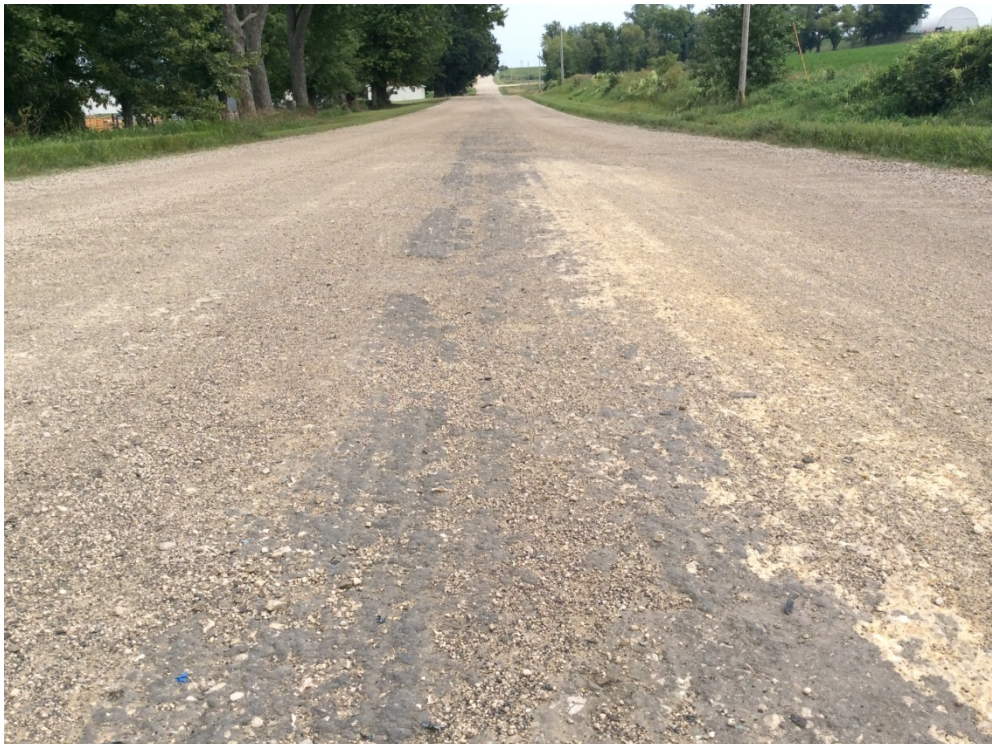
Figure 11. Close-up shot of TOSS LS CL6 2013 Section facing east
